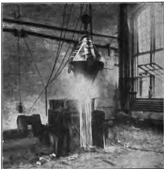
FIG. 95.—Thermit crucible as used for welding.
